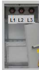
Figure 26 – Marking of the phases
